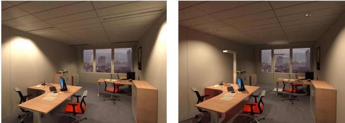
Figure 4: Example of two lighting installations in an office, using ceiling mounted circular luminaires, and task lamps. Left, with fluorescent, and right with LED solutions. LED solution is 50% more energy efficient, but LCC is lower only with long life LED systems.
